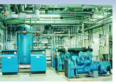
The V-Compact is a free standing, single acting, lubricated or oil free unit set on anti-vibration mounts and is suitable for air or water cooling. Pressures range from 1.5 to 10.5 bar g, and power from 18 to 63 kW.
